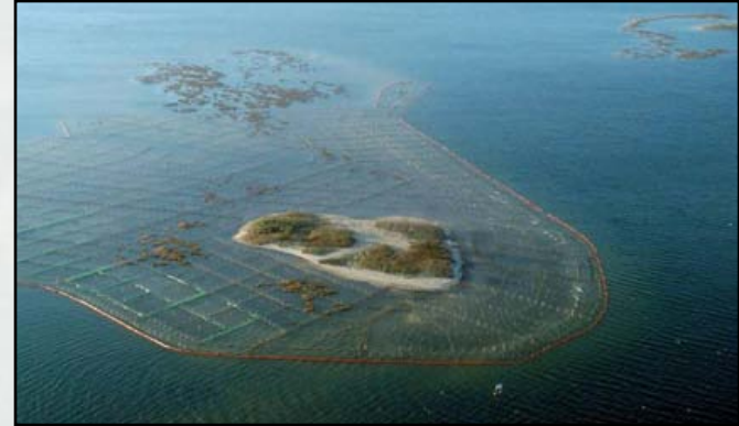
Restoration work in Jamaica Bay, NY
