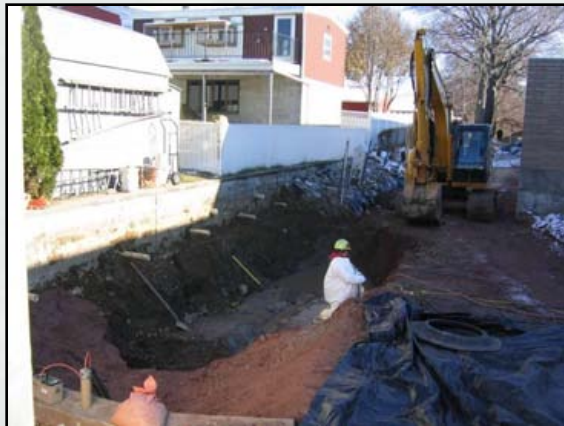
Ongoing FUSRAP work in Maywood, NJ
