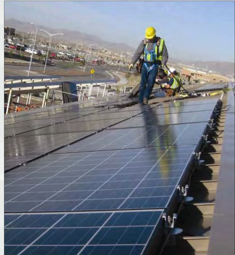
The Brigade Combat Team Dining Facility at Fort Bliss, TX, is powered by solar panels.
